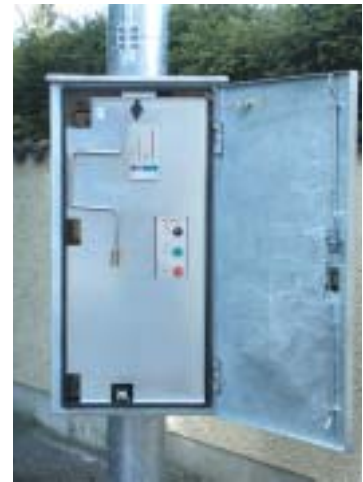
Example 2: control unit with mounted motordrive UM20 for radio control
